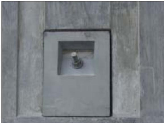
Fig. 21 Anchor plate installed in the precast retaining wall
