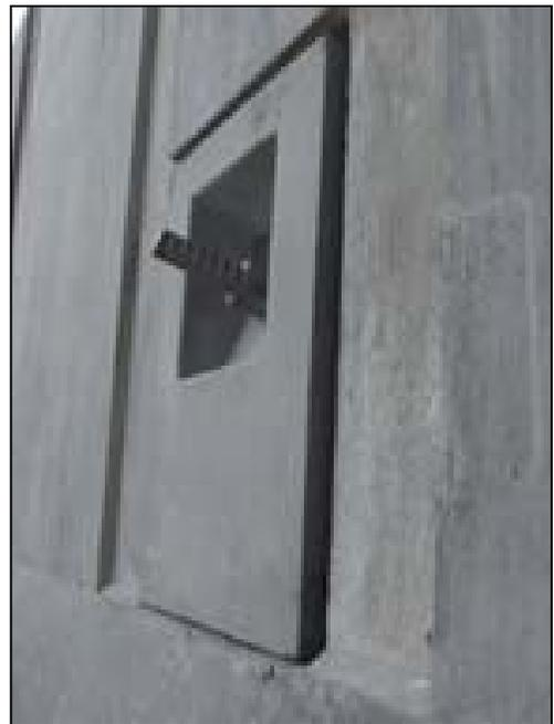
Fig. 22 Anchor plate installed, elevation view
