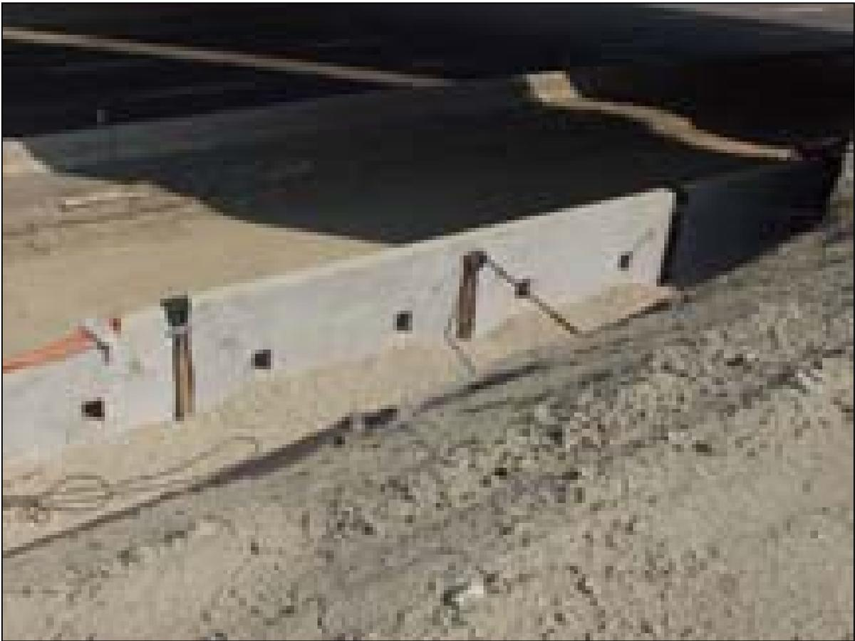
Fig. 18 Precast retaining wall
